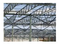
The Open Web Bar Joists serve large segment of construction industry especially the roof systems for single story retail buildings. Roof systems made with open web bar joists are extremely popular because of low cost and quick construction. Information about the steel joists can be obtained from <a href="https://www.steeljoist.org">www.steeljoist.org</a>. This website offer many free publications, videos and CAD drawings to understand steel joists and the
