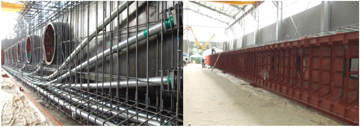
Figure 4: Reinforcement and Formwork
