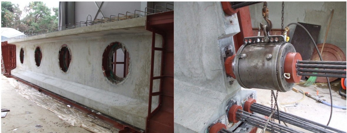
Figure 5: Demolding and First Stage Prestressing
