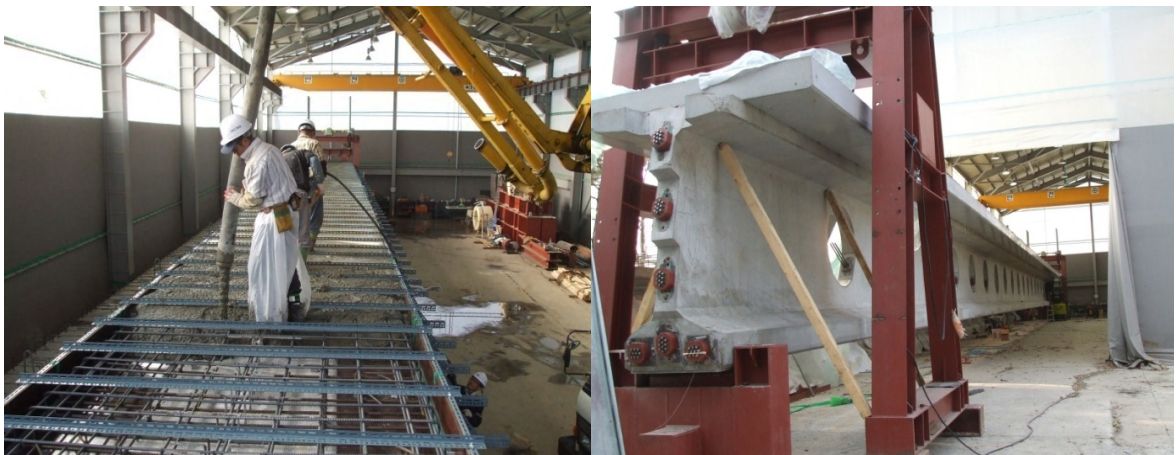
Figure 6: Deck Slab Casting and Final Appearance
