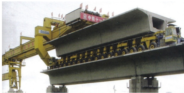
Figure 2: Prefabrication method with transport of the segments on the section constructed
